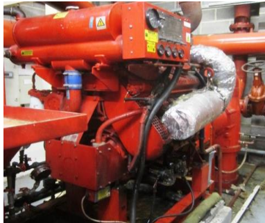
Detroit Diesel Fire Engine pumps (3-off)
