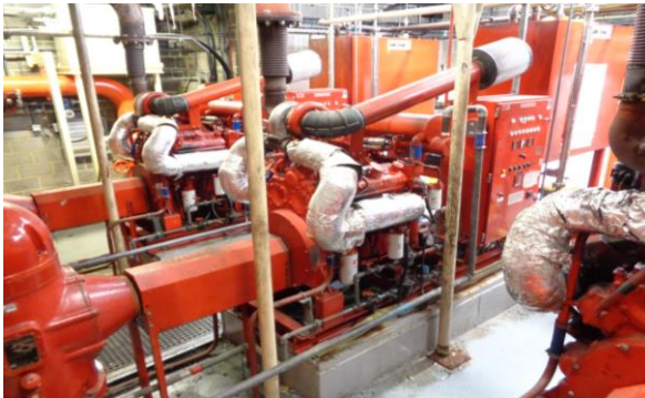
Detroit Diesel diesel fire engine pumps (3-off)
