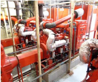
Detroit Diesel Fire Engine pumps (3-off)
