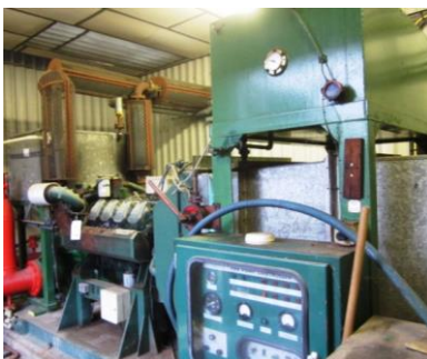
Sigmund Pulsometer fire engine pump with Fiat engine (2-off)
