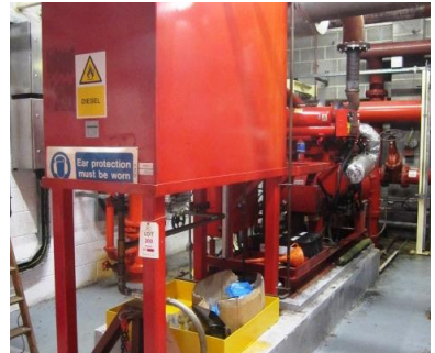
Detroit Diesel Fire Engine pumps (3-off)
