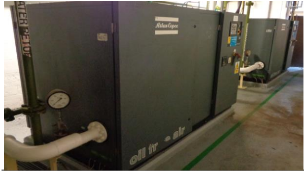
Atlas Copco ZR145 compressors (3-off)
