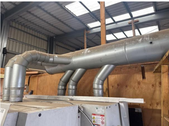
Bale-Pak dust extraction trunking/system
