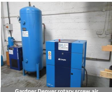
Gardner Denver rotary screw air compressor, model L22 RS (2022), air receiver, Dry Point RA air dryer
