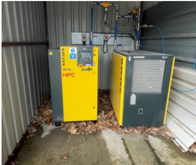
HPC SK25 rotary screw compressors (3-off)
