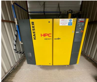
HPC BSD 75T & ABT 60 rotary screw air compressors (2-off)
