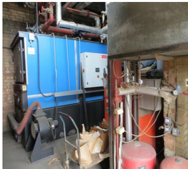
Ran Heat Biomass boiler
